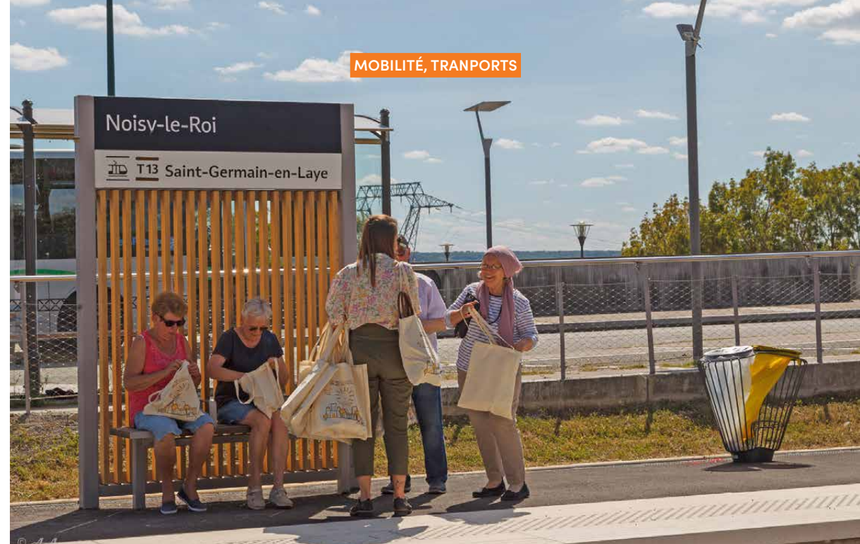
Station de tramway, Noisy-le-Roi.
